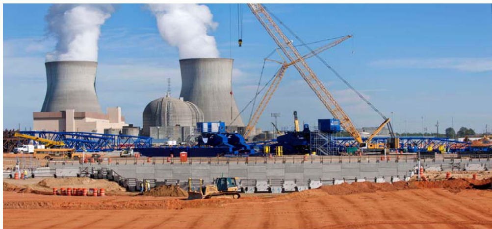
FIGURE 2.13 New construction at an existing two-unit nuclear power plant. SOURCE: © Southern Company, http://www.southerncompany.com/nuclearenergy/photos.aspx . 1
