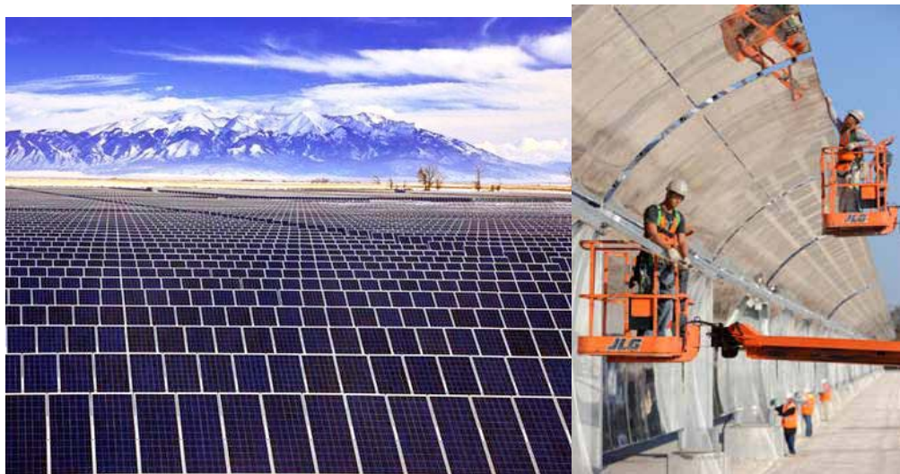
FIGURE 3.1 ( Left ) Utility-scale PV system . ( Right ) Construction of concentrating collectors for the Martin Solar Plant (a concentrating solar power system). SOURCE: ( Left ) http://solarpanelspower.net/solar-power/the-politics-of-solar-power . ( Right ) Sherwood (2011).
