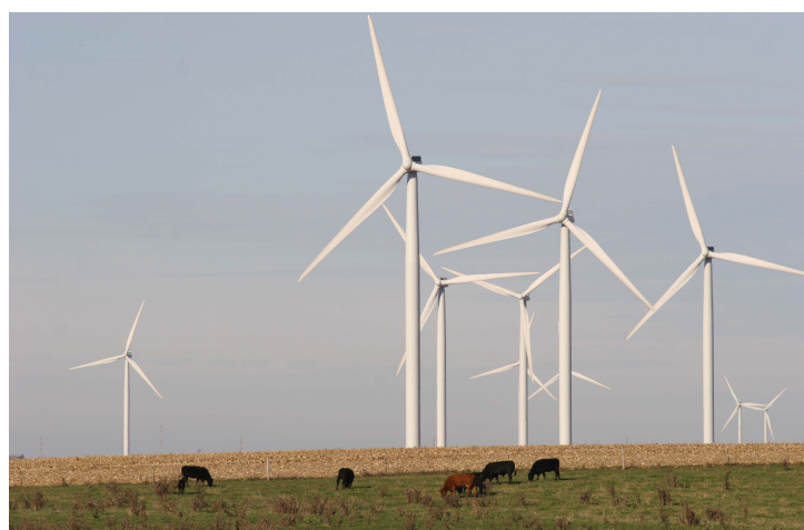
FIGURE 3.6 Wind farm. SOURCE: http://www.dis.anl.gov/projects/windpowerforecasting.html . Used with permission from U.S. DOE’s Office of Science.
